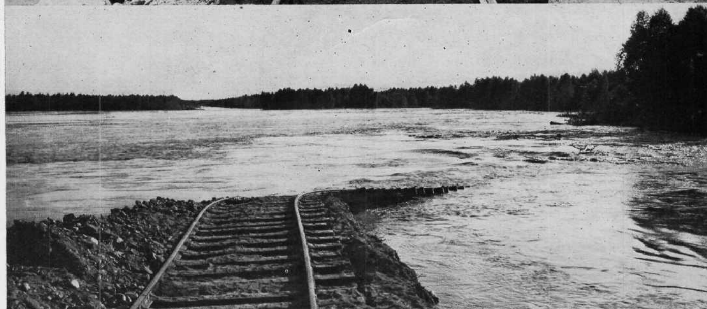
When Imperial Valley was reclaimed, rock-reveted levees were built along the west bank of the Colorado to keep flood waters from breaking through and inundating the basin. The two pictures above, taken from approximately the same point, show how the mighty power of the river occasionally breached these levees. Photos by Hetzel, El Centro.
